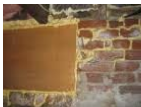
Air seal foundations with foam
