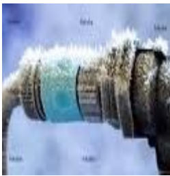
Garden hose left connected can cause inside leaks
